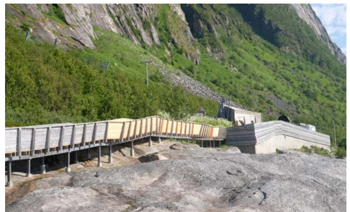
Viewpoint Tungeneset by Code, under repair. (Photo credit: Jordan Silver)
